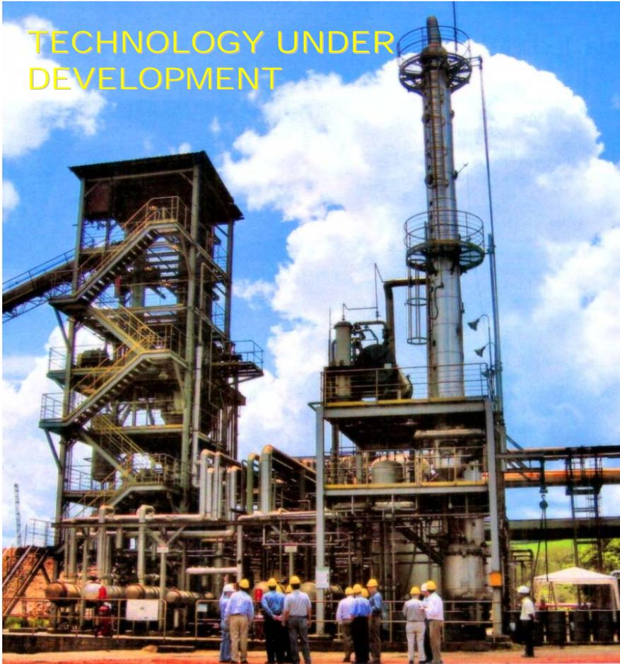
REACTOR TOWER. DISTILLATION PRODUCTS RECOVERY EQUIPMENT: HYDROLYSED LIQUOR, RECOVERED SOLVENT (ETHANOL), LIGNIN, HYDROLYSED LIQUOR TREATMENT AND MIXING WITH TRADITIONAL MASH (FROM SYRUP/MOLASS)
